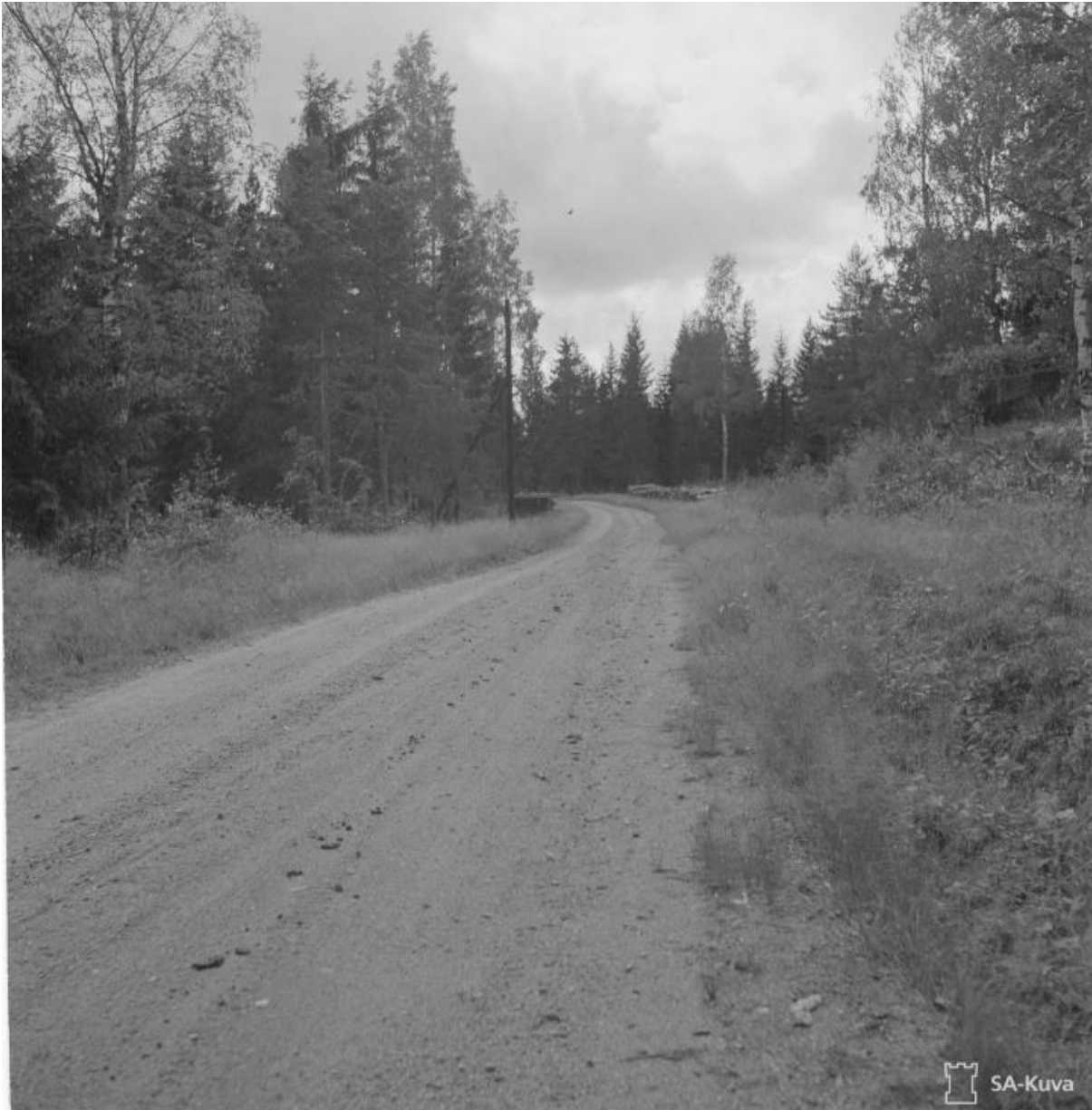
A typical Karelian road and typical woods (SA-Kuva)
